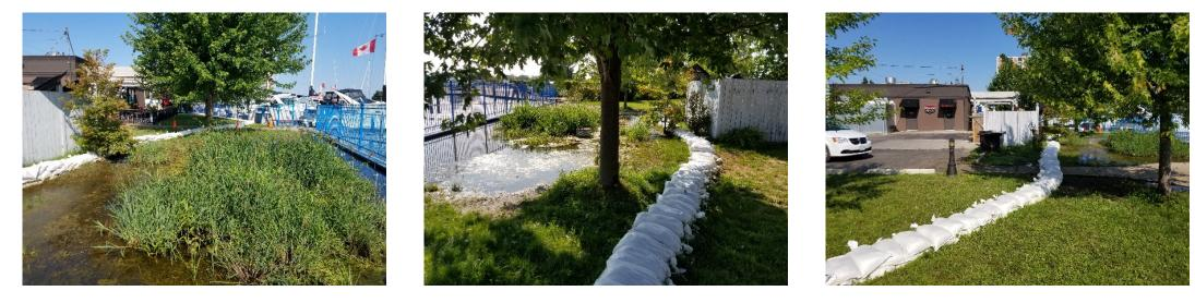
**LAKEVIEW MARINA** – Water level elevation of 175.6m on Aug 2<sup>nd</sup>. Observed pooling of water in the area between Armando's Pizzeria and the sheet piles boundary of the marina. Sandbagging in place limits flooding to this immediate area, but if allowed to flow freely, overland flow at this location would reach Riverside Drive and flow down Riverdale Ave.
