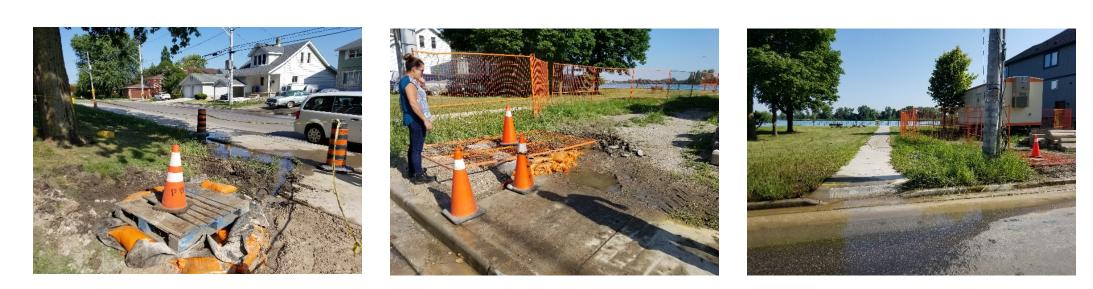
**8717 RIVERSIDE DRIVE** – Water level elevation of 175.6m on Aug 2<sup>nd</sup>. Observed water flowing onto Riverside Drive from storm sewer manhole. This manhole is connected with outfall from 8717 Riverside Drive to the Detroit River.
