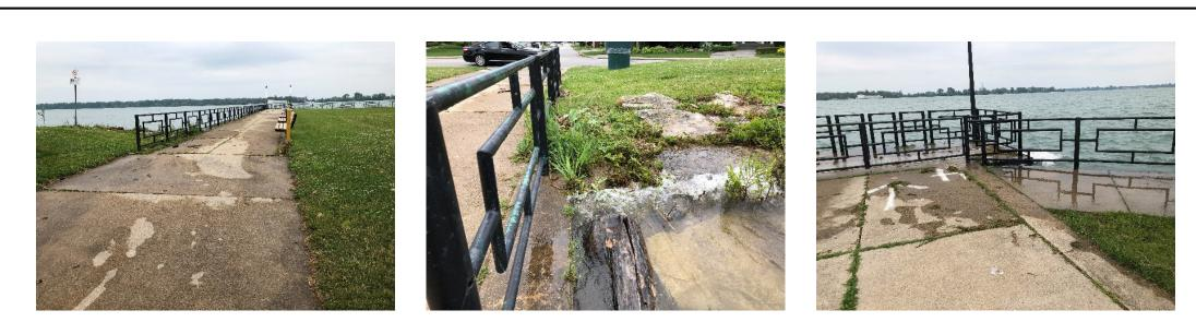
**ST. ROSE BEACH** – Water level elevation of 175.7m on July 7<sup>th</sup>. Observed shallow waves overtopping pedestrian walkway and spilling water and debris onto Riverside Drive.
